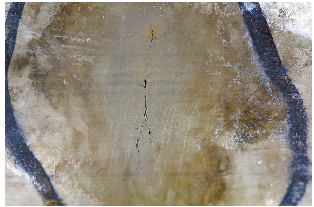
Fig. 2: Detail from image 1: place of damage with crack field \approx 3:1
